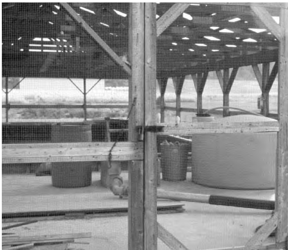
Figure 2. Secure and disable tanks to prevent unauthorized access.
